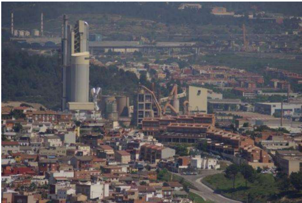
Figure 5 Image of Sant Vicenç dels Horts in the foreground and the cement factory in the background, in the same municipality.
